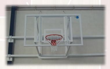
The basket cantilever is 2,25 m; however, they can be adapted to the particular conditions of each installation depending on the court situation respect to the fixing point of the basket.
